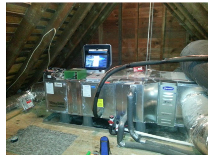
The Unico System ECM Software being configured via laptop
