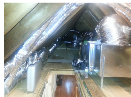
The Unico System and ductwork installed in attic
