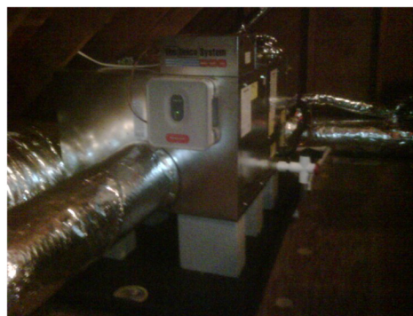
The Unico blower and coil with the ACB in the attic
