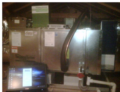
The Unico Green Series being programmed via laptop
