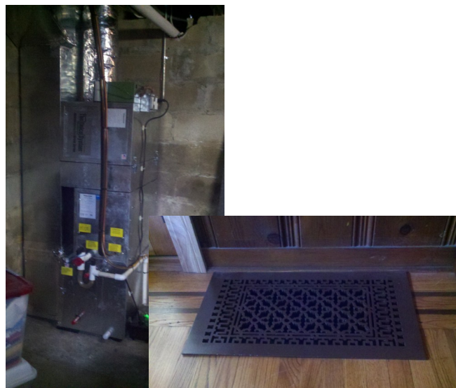
Unico EC blower and coil in the basement and a custom made return grill
